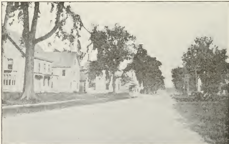
Main Street, North Windham, Maine
